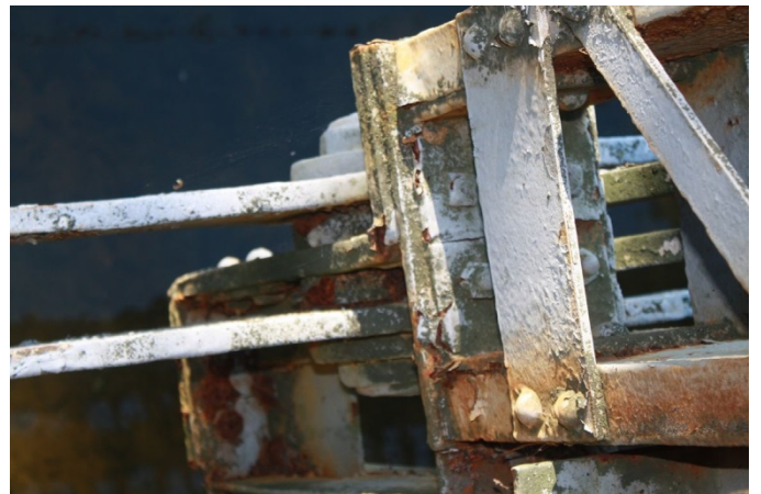
Lower chord connection (typical).
