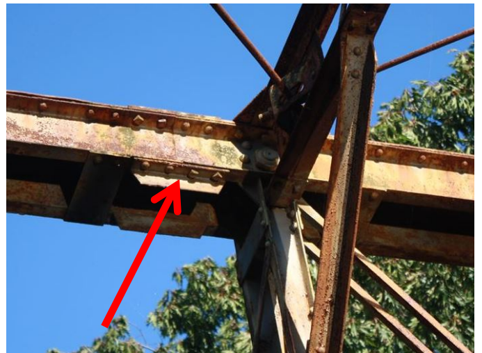
Section loss at base of vertical member.
