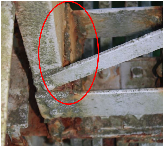
Pack rust and section loss at base of vertical member.
