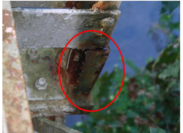
Section loss at base of vertical member.
